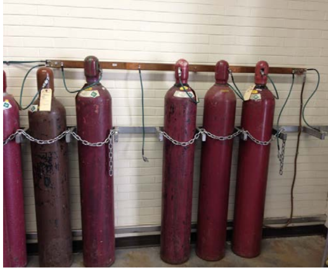
Figure 8: Compressed gas cylinder storage area. Image courtesy of Safety Resources.
