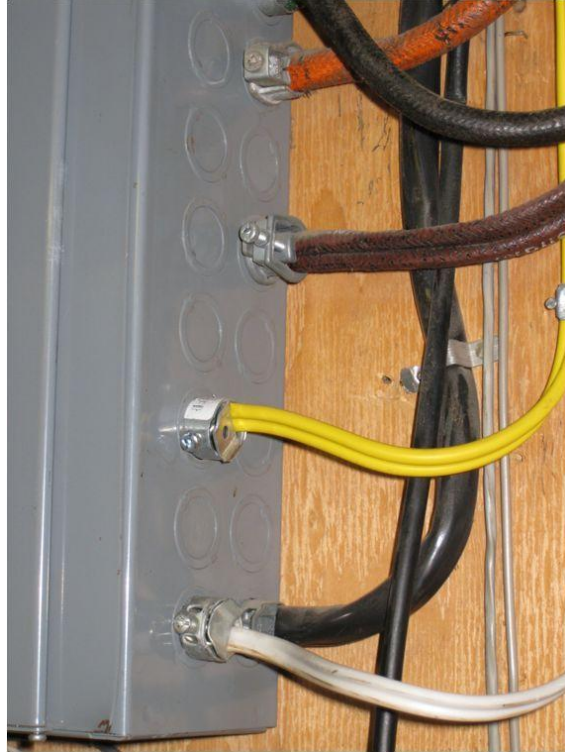
Figure 6: Example of cable clamping and grip devices. Image courtesy of University of Saskatchewan.
