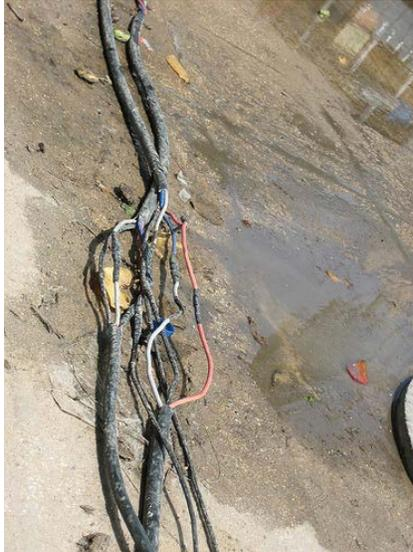
Figure 4: Frayed wires and power cables pose a significant electrical hazard. Image courtesy of marblegravy, Flickr.
